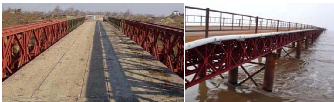
Figure 6. Illustrations of temporary Bridges
