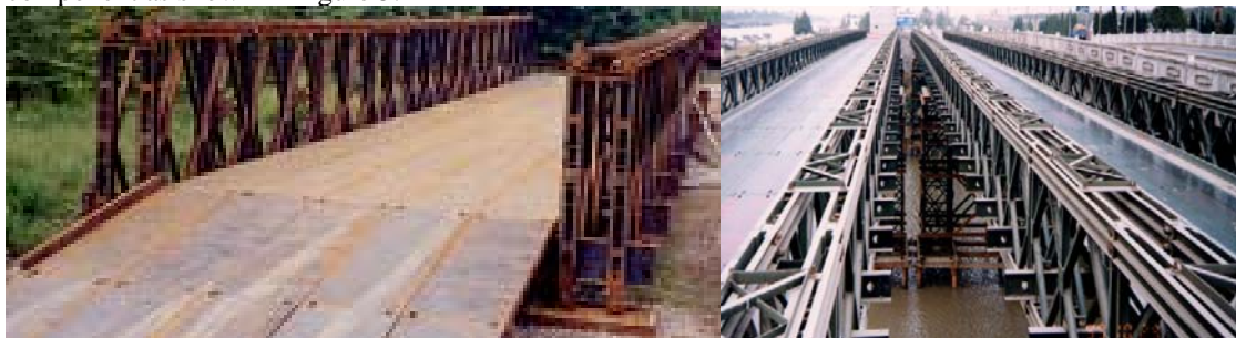
Figure 5. Illustrations of Prefabricated Highway Steel Bridge (PHSB)
